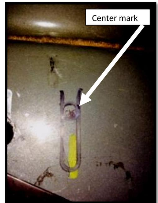
**Step 6:** Remove clip. Use a 1/2” drill bit and drill out the center mark. Slide the 3/8 clip back into position so the threaded part is aligned with the hole.
